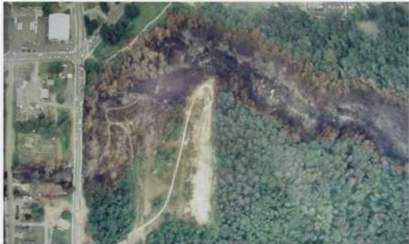
Figure 4-16: Aerial photo of damage area from 1999 Bellingham Olympic Pipeline rupture and fire. The rupture occurred upstream to the right of the photo. Resulting fire extended several hundred feet on both sides of creek.
